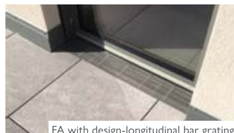
Slot top with drainage-slots for drainage of the second level
